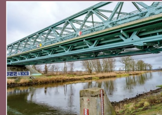
Most na Noteci Netzebrücke
